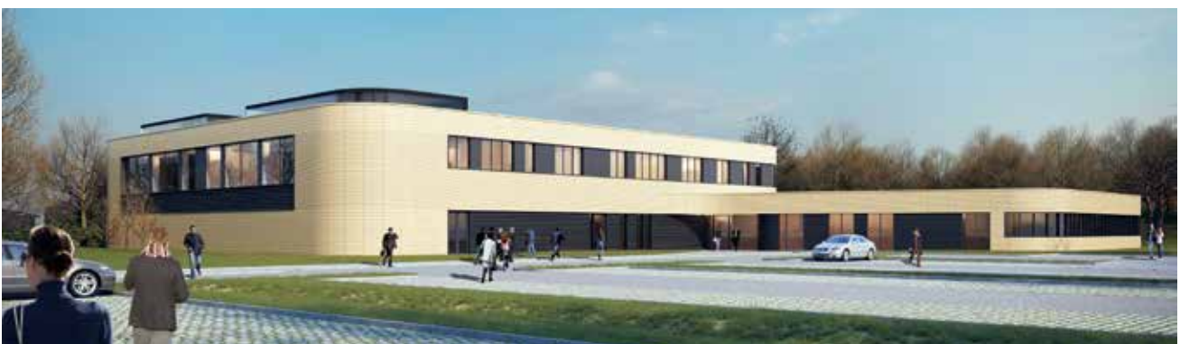
North Harrislee control center
